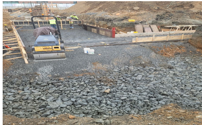
Nyack Hospital parking Garage footing
