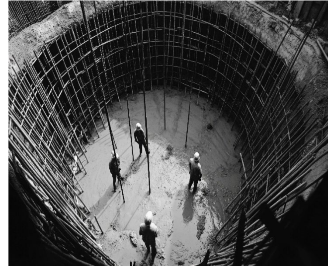
cylindrical reinforced concrete foundation
